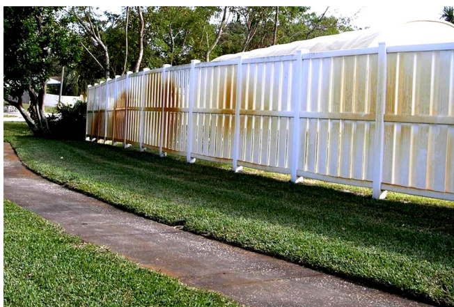
Figure 12. Iron stains on the fence show the use of an irrigation radius that is too large for this area Credits: Bryan Unruh
